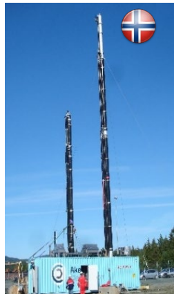
Natural gas Risavika Gas Center
