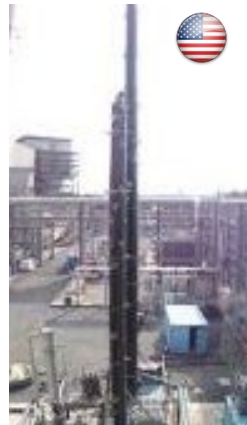
Coal National CCC
