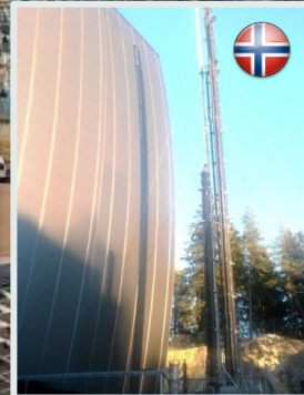
Waste to Energy Klemetsrud WtE
